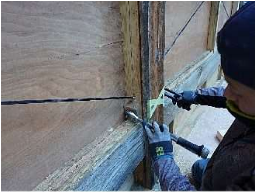
Photo 5: Control of tightening torque
