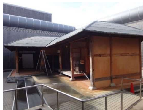
Photo 1: Appearance of the target building (Before reinforcement)
