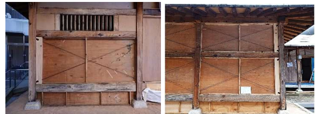
Photo 3: Appearance of the target building (After reinforcement)
