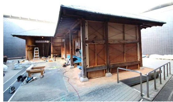
Photo 2: Appearance of the target building (After reinforcement)
