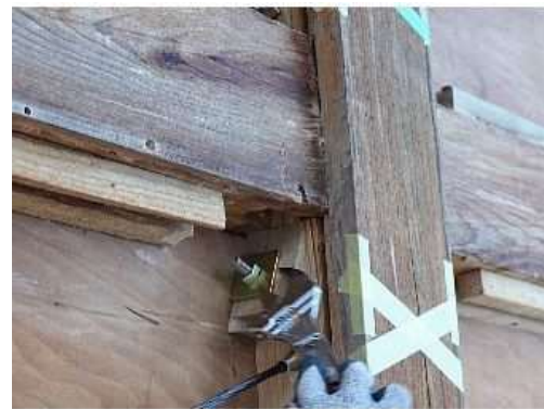
Photo 4: Control of tightening torque
